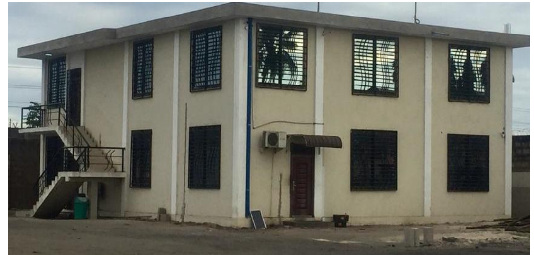
Office Block & Workshop, Dar Es Salaam
