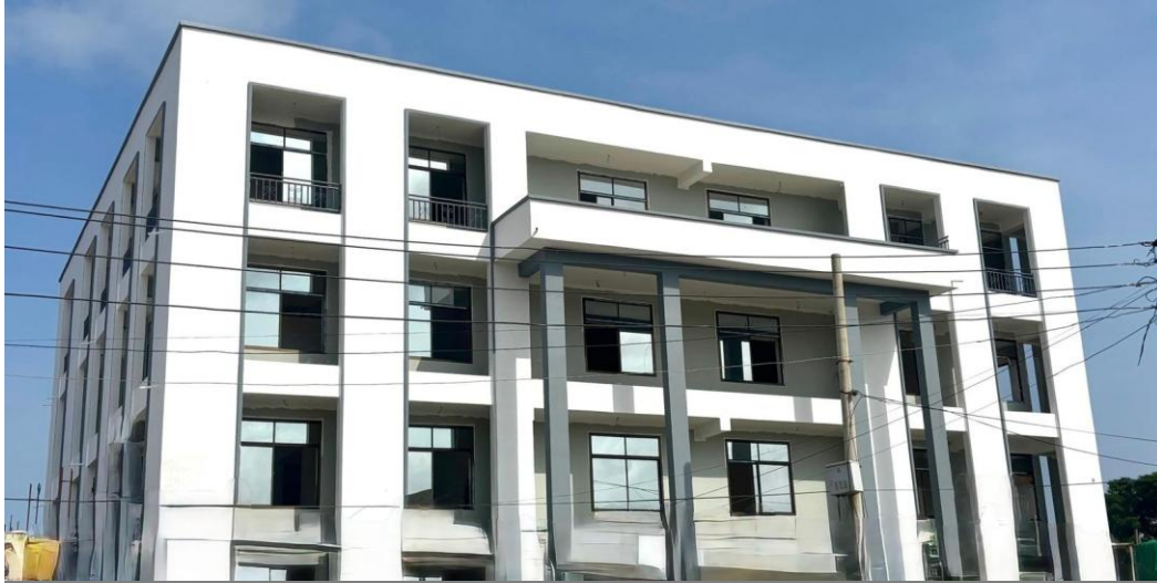
4 storey orphanage building, Dar Es Salaam
